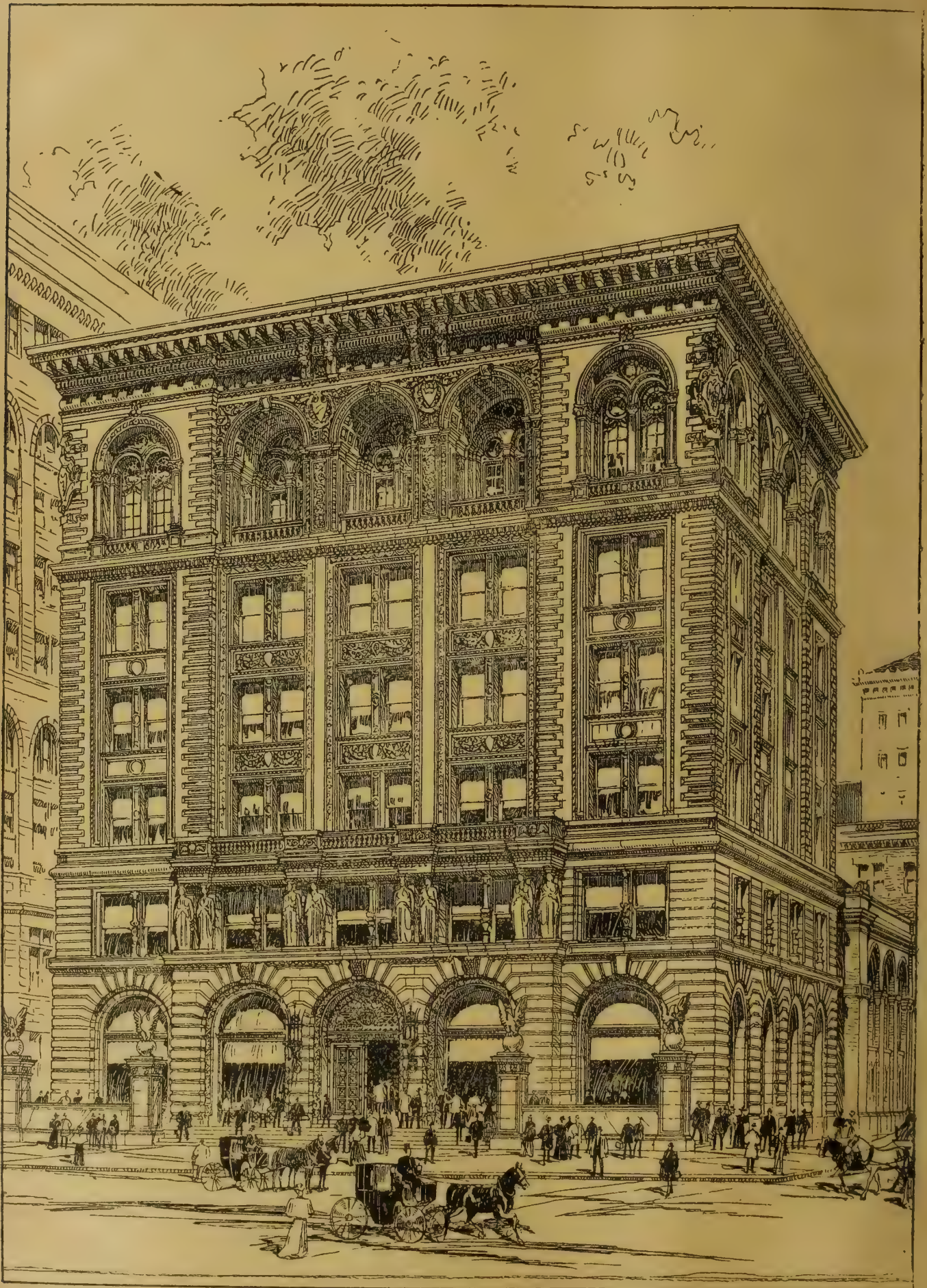
CHAMBER OF COMMERCE BUILDINGS, CLEVELAND, OHIO.
